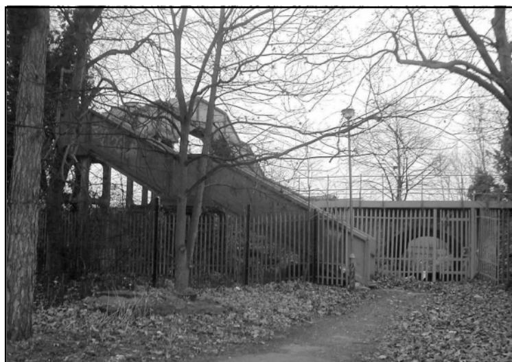
The old concrete bridge has now been removed.
