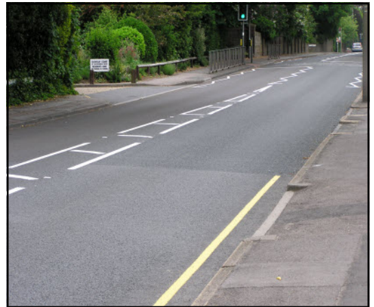
The centre white lines were put back straight away after resurfacing but not the yellow lines at the side
